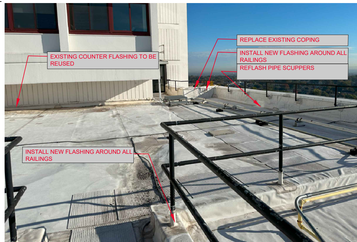
2 EXISTING CONDITION PHOTO NTS
