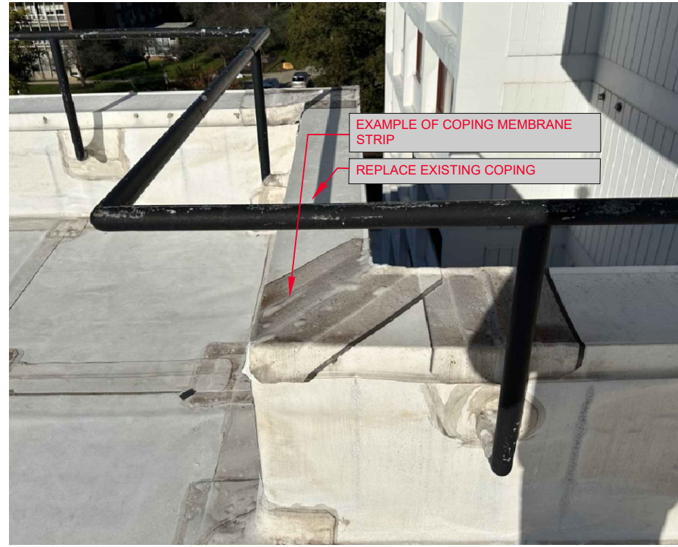
5 EXISTING CONDITION PHOTO NTS
