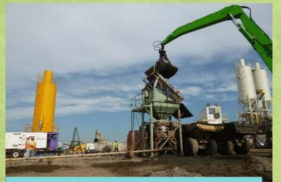
a) Grizzly/vibrator, screen, and mixing plant
