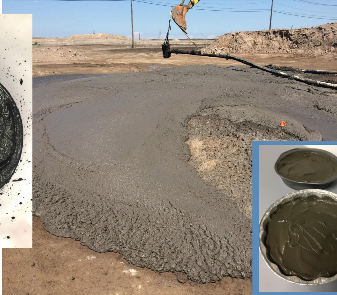
Freshly-placed PFTM Processed Sediment (8% Portland cement)
