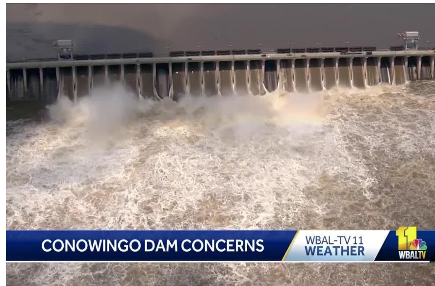
Conowingo Dam overflow event
