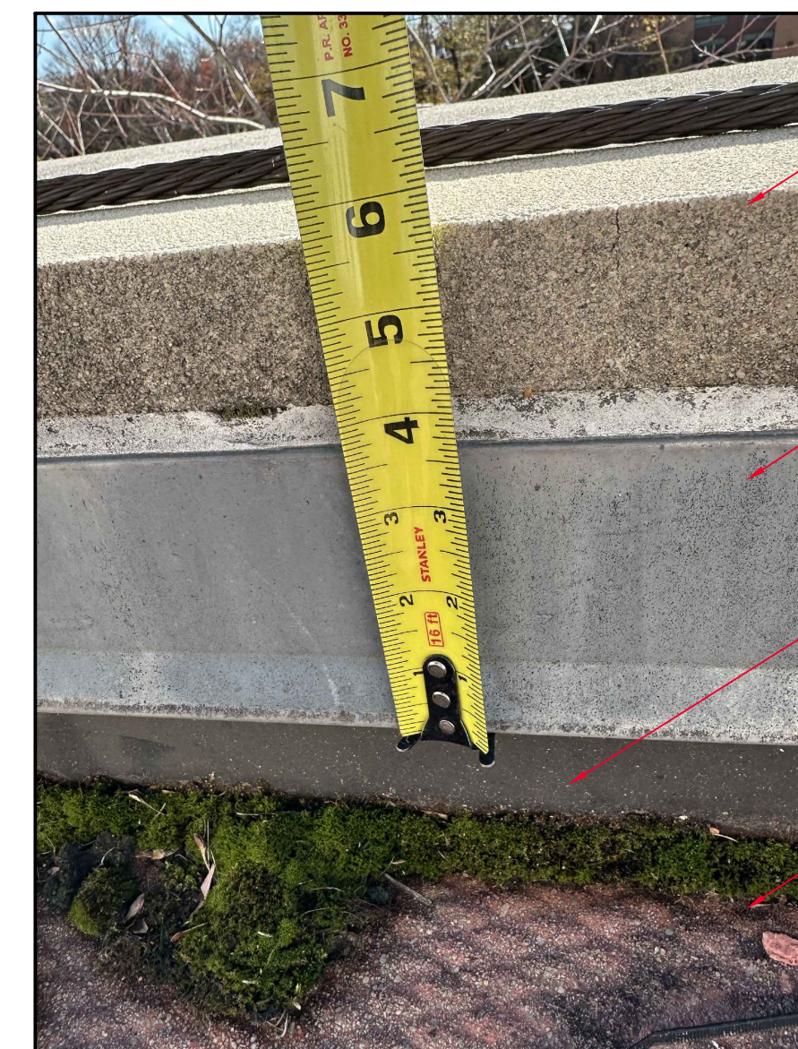
PARAPET FLASHING
