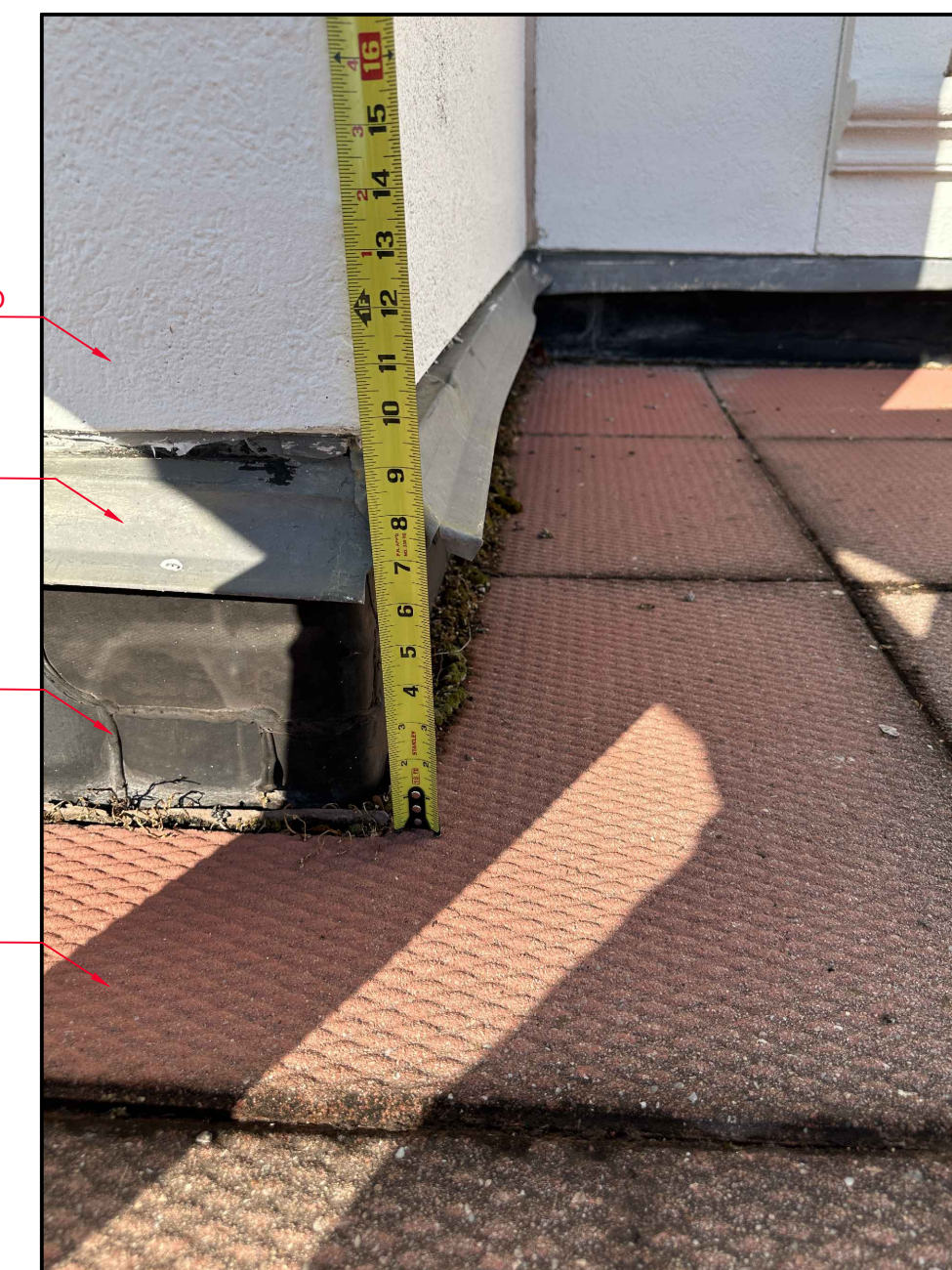
BUILDING WALL FLASHING
