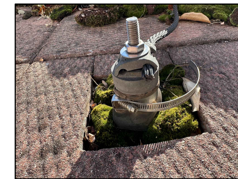
LIGHTNING PROTECTION PENETRATION
