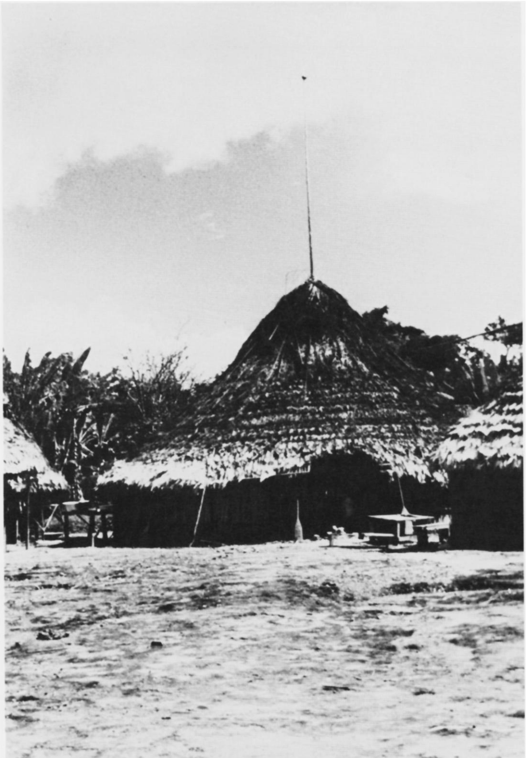
Figure 3. Form of the traditional communal round house ( müimó ) constructed by the Waiwai. This particular structure (2E in Figure 2) is nearly 10 m in diameter and houses six individuals.
