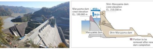
Figure 3-9 Dam upgrading (relocation) experience in Japan: Replacement of Ōyubari with larger Yubari Shuparo (left image – received from Y. Shimizu) and the Maruyama dam upgraded by Shin-Maruyama (right plot - https://doi.org/10.20965/jdr.2018.p0585)
