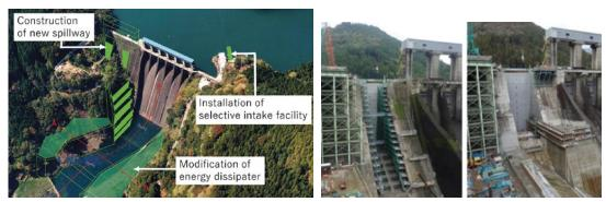
Figure 5-15 Example of intake and discharge facilities modification at Nagayasuguchi dam (Sasaki and Kondo, 2018)
