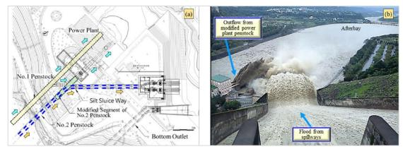
Figure 5-4 Modified segment of second penstock being used for sluicing and flushing (left drawing) and sediment sluicing through modified penstock and spillway (right image) during the first operation in 2013 Typhoon event (Lee et al., 2022)
