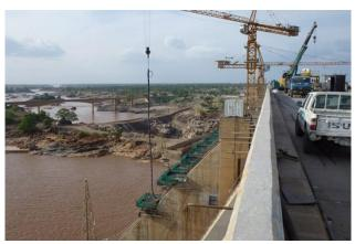
Figure 5-20 Heightening of Roseires dam (http://pf.bbrnetwork.com/)
