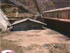
Figure 3-20 Sediment deposited in (left) and around the powerhouse (right) as a result of a sediment hazard during flushing operation at Pillur reservoir in India (Giri et al., 2019)
