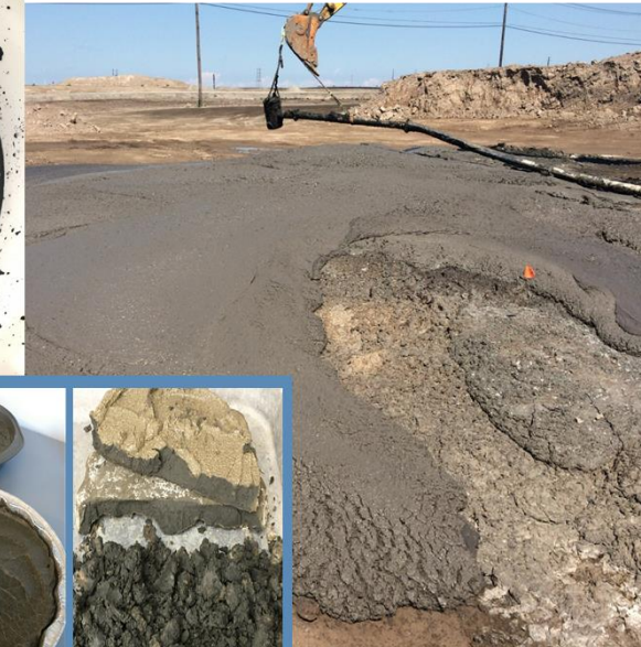
Freshly-placed PDM (8% Portland cement via Pneumatic Flow Tube Mixing)
